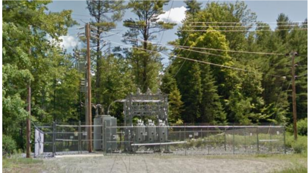
Typical Substation at point of interconnect – located on site adjacent to transmission line
